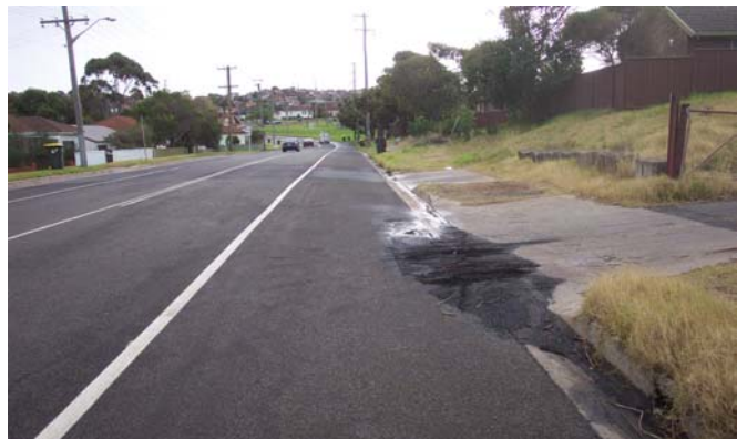
Looking north along the on Road cycle lane on Shellharbour Rd
